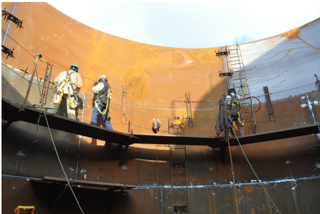
Workers weld seams in hydrolysate storage tanks
