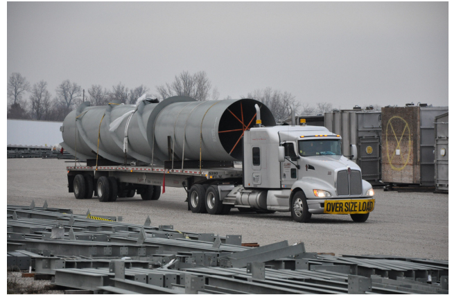
Clean air exhaust filter stacks being moved through a lay down area
