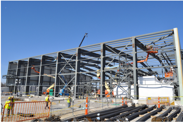
Structural steel progressing at Super Critical Water Oxidation (SCWO) processing building
